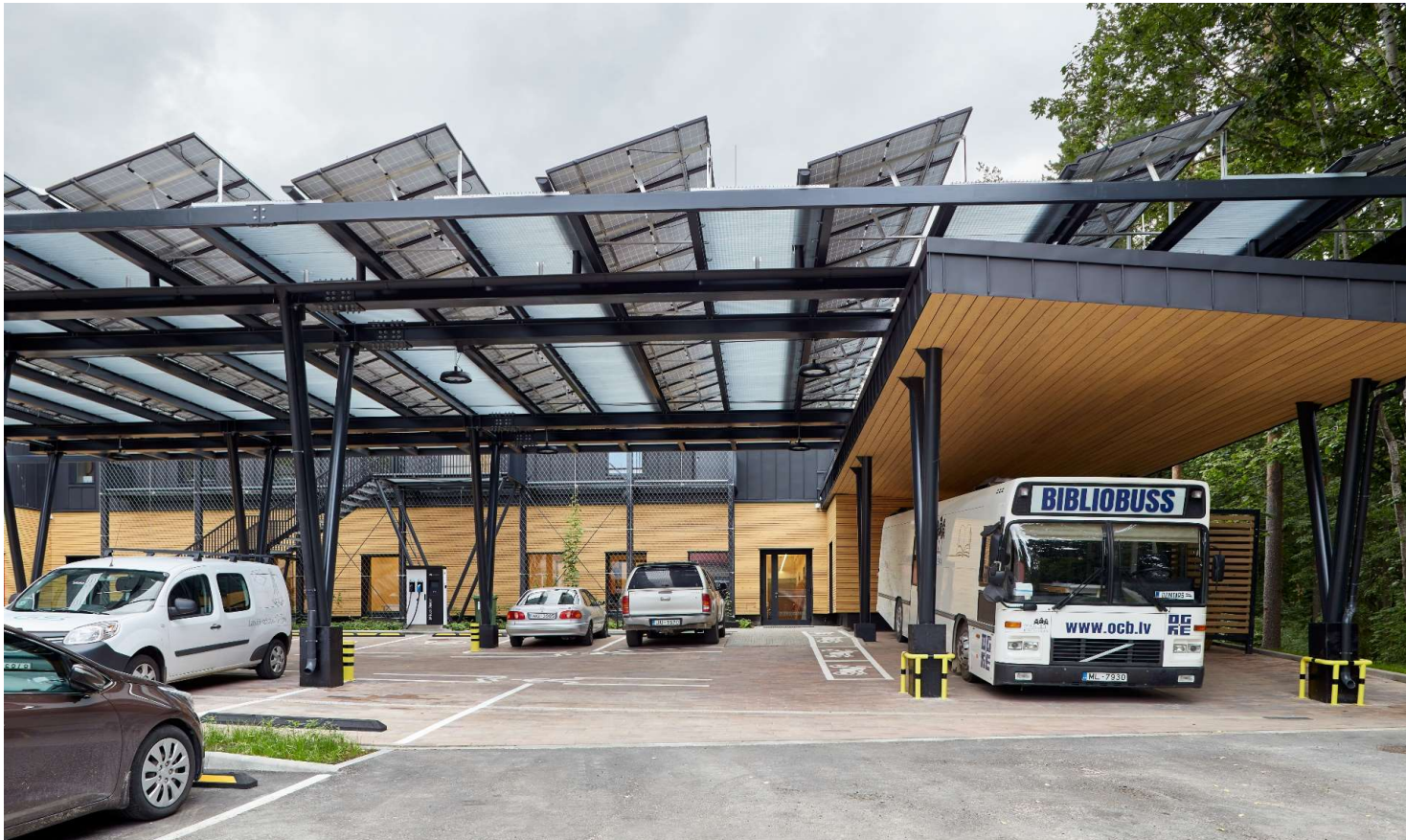
SOLAR PANELS 117 CAR CHARGING STATIONS 2
