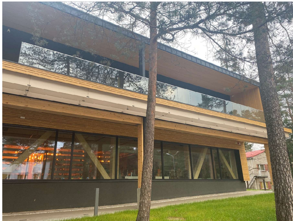
1. THE OVERHANG OF THE 1 ST AND 2ND FLOOR COVERINGS ON THE SOUTH SIDE
